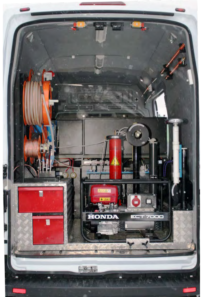
View of the High Voltage area
