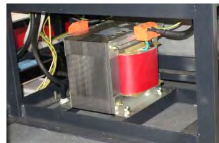
View of Isolation Transformer
